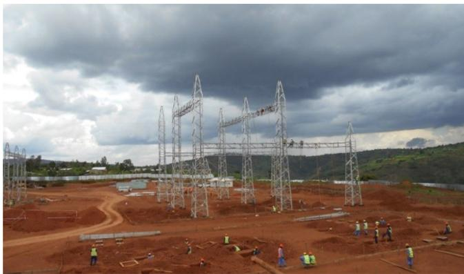
Figure 1: Shango Substation Under construction- Rwanda
