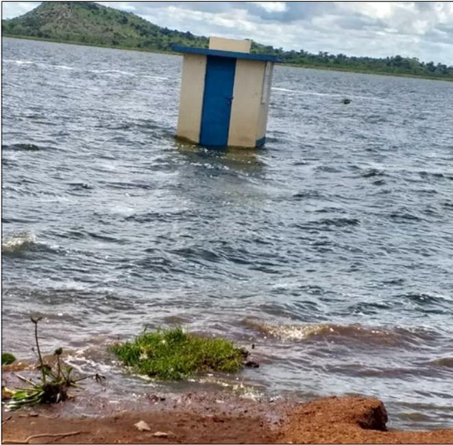
Fig. 4. Submerged hydro-met station around Lake Kyoga, in Uganda.
